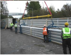
When fully assembled the Pack Boy<sup>™</sup> is capable of lifting rigid packs of panels up to 20m long and weighing up to 4 tonnes.
