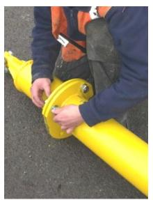
Lay out the beam struts end to end in the correct configuration, using the flats on each flange to prevent rolling. There are 3 x 2m beam struts on top of the stillage with a 1m strut and two end sections inside the stillage.
