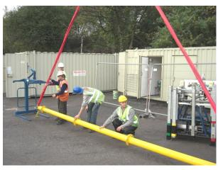
Once the beam is fully assembled in the correct fashion, attach one lifting sling through each of the large top shackles, ensuring that the shackle pin is securely tightened afterwards.
